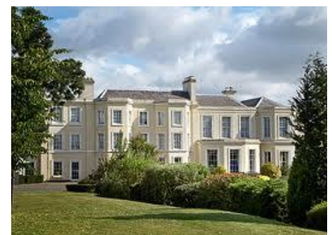
The Burnham Beeches Hotel
